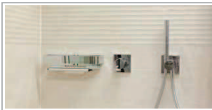
CONCEPT BAU – CITY LOUNGE – Detail Bad
